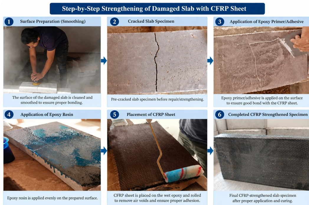
FIGURE 3.3: step by step strengthening of BC slab
