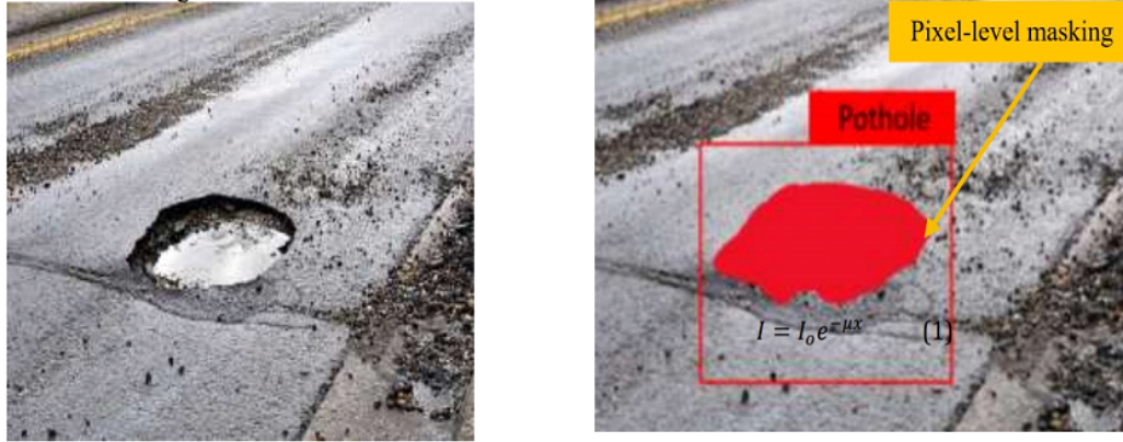
FIGURE 2.11: YOLO 8v-seg bounding box and pixel-level masking of pothole [90]
