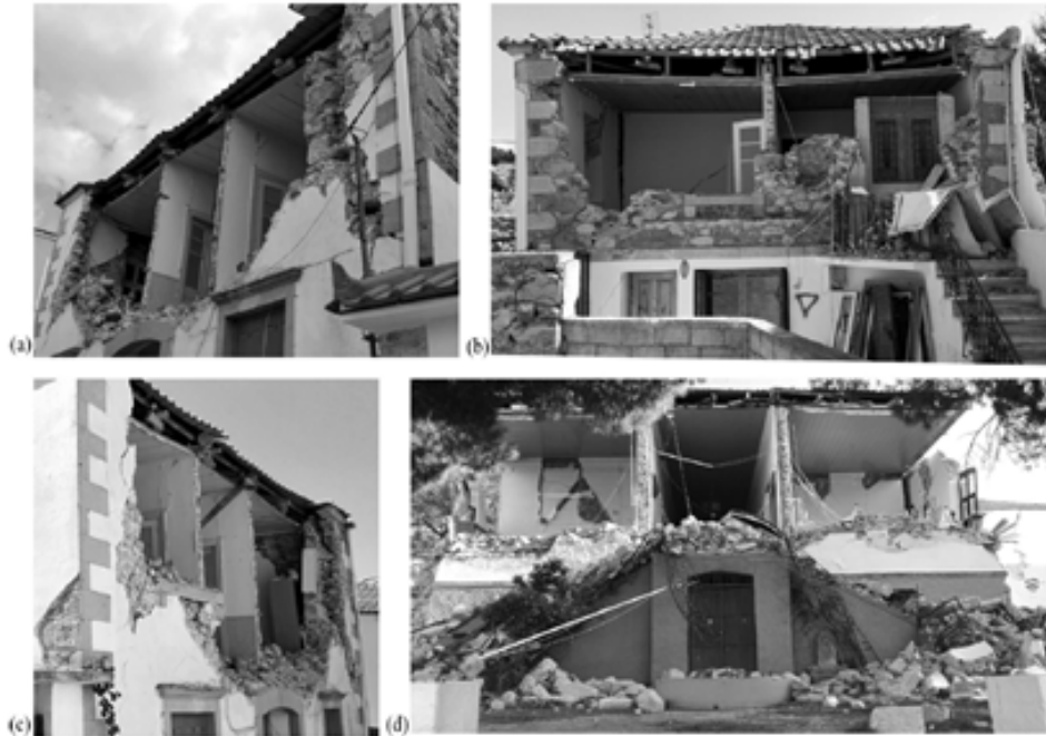
FIGURE 2.1: Typical out-of-plane failures of conventional masonry under one-way and two-way bending [1].
