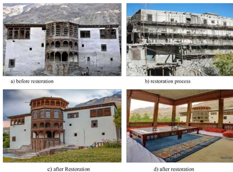
FIGURE 2.3: Photographs show Khaplu Fort restoration.
