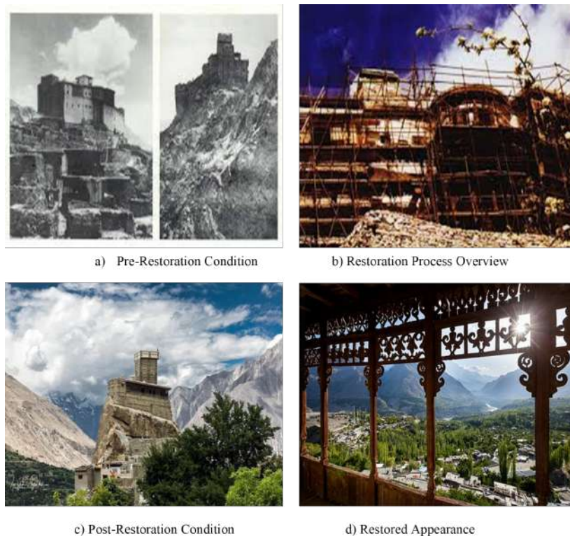
FIGURE 2.1: Photographs of Altit Fort restoration
