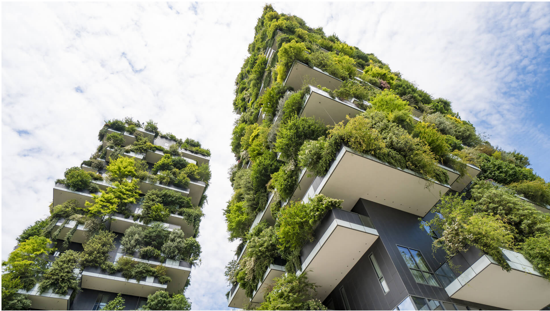
FIGURE 1.1: Bosco Verticale (Vertical Forest), Milan – a model of sustainable high-rise architecture integrating over 900 trees and 20,000 plants on its facade, enhancing biodiversity, air quality, and energy efficiency [16].
