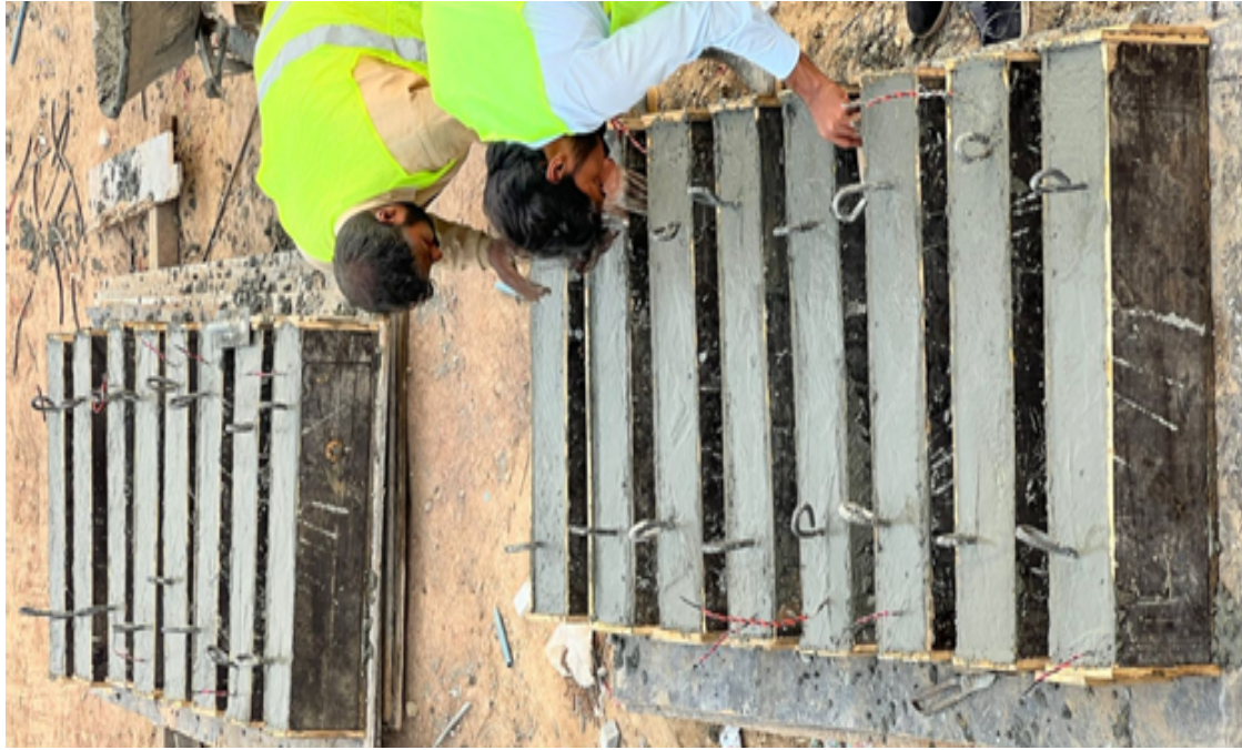
FIGURE 3.16: All Beams after concreting and surface leveling
