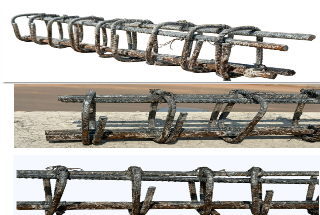
FIGURE 3.45: Extraction of corroded steel skeleton
