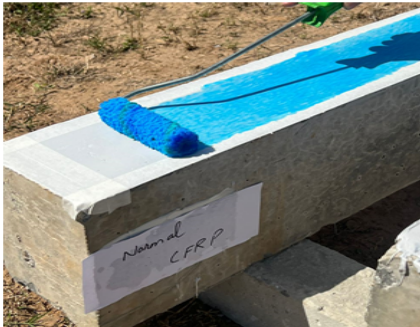
FIGURE 3.28: First coat of adhesive
