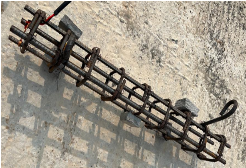
FIGURE 3.9: Beam steel skeleton longitudinal face
