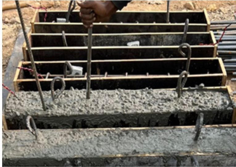
FIGURE 3.12: Manual Roding to remove air voids
