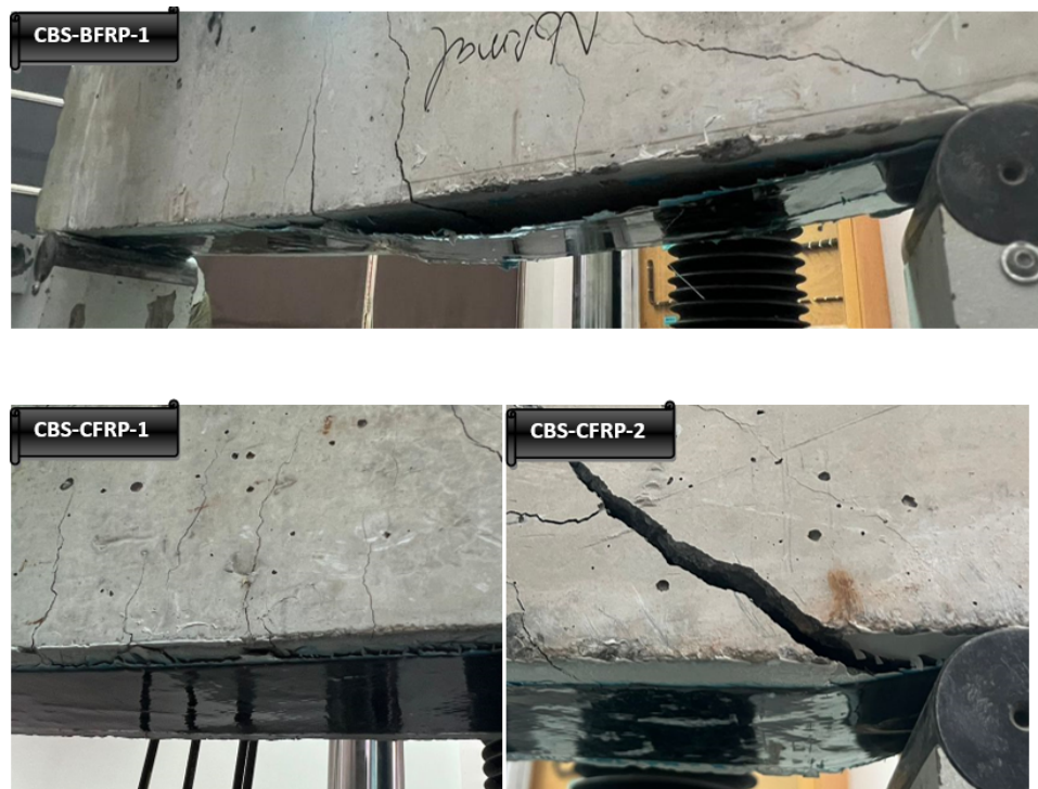
FIGURE 4.11: Adhesive failure and de-lamination
