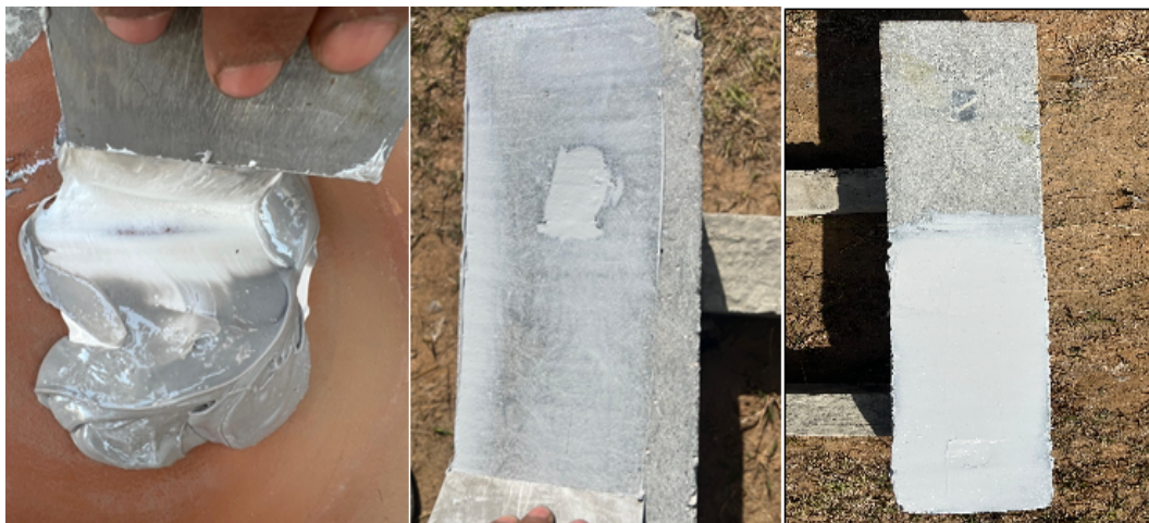
FIGURE 3.24: Base Epoxy mixing and application
