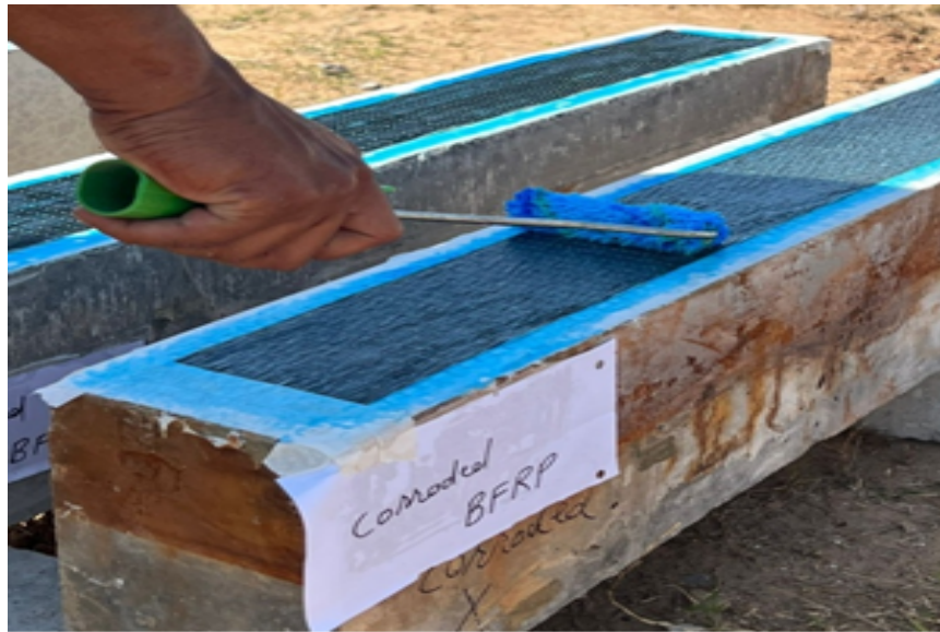
FIGURE 3.30: Final coat of adhesive
