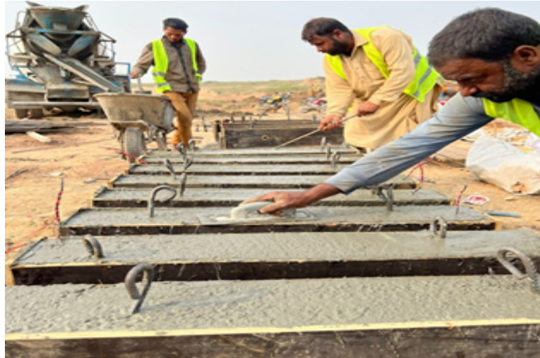
FIGURE 3.14: Surface troweling &amp; Leveling
