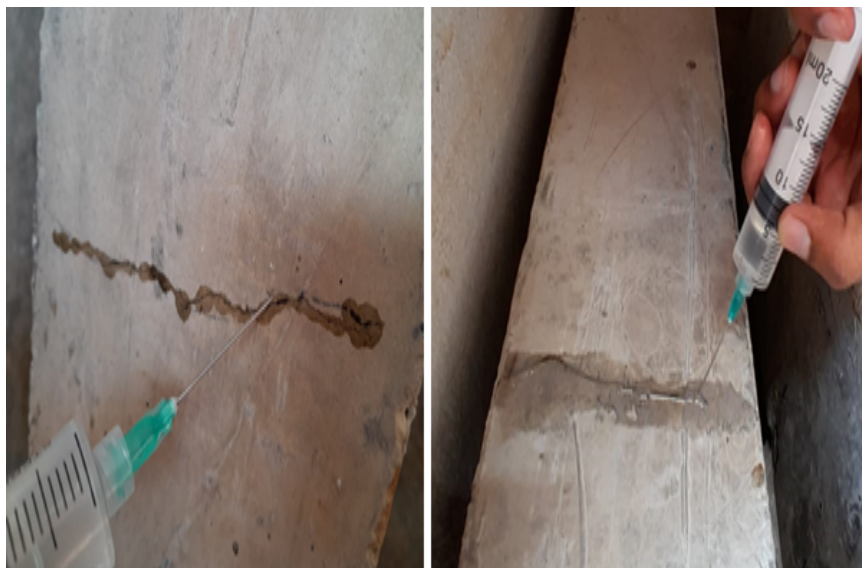
FIGURE 3.32: Cracks filling with filler resin using injection
