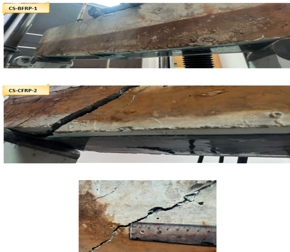
FIGURE 4.10: Laminate tear out at mid span, at supports, and 0.5cm cracks
