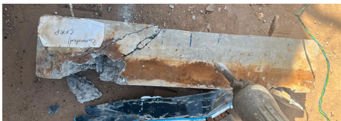
FIGURE 3.44: Extraction of corroded steel using hilti
