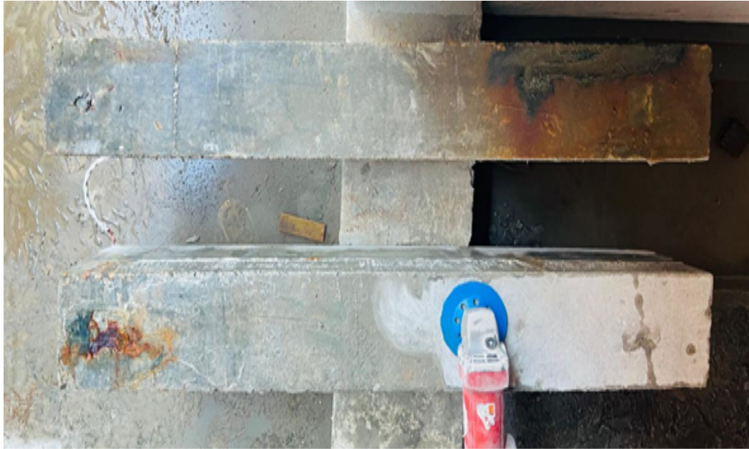
FIGURE 3.23: Beam soffit surface grinding
