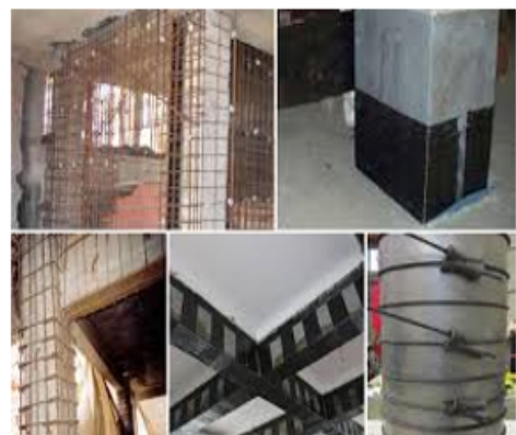
Fig d): Strengthening using CFRP & BFRP laminates
