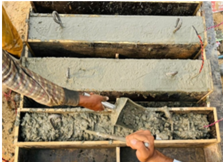
FIGURE 3.13: Scoop to pour concrete from TM
