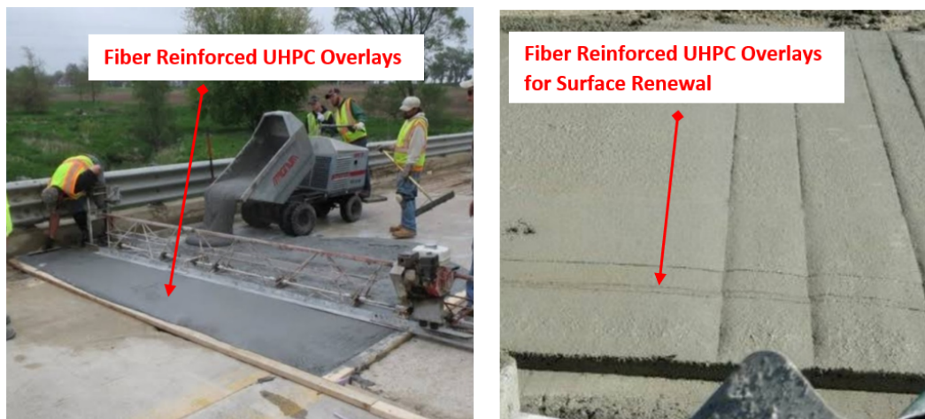
FIGURE 2.10: Fiber Reinforced UHPC overlay [50].
