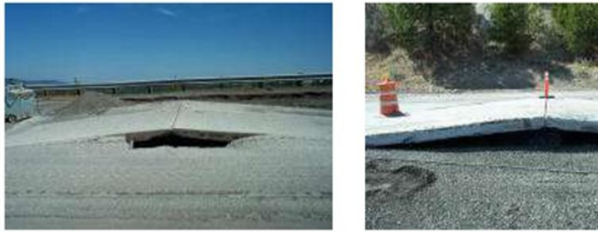
FIGURE 2.5: Severe Blowup [12].
