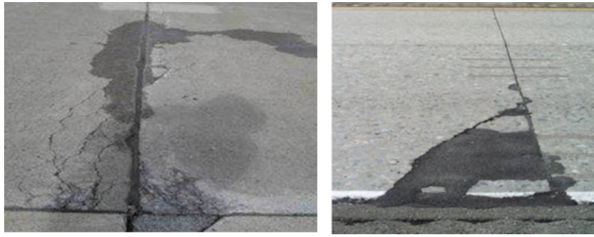
FIGURE 2.6: Joints Deterioration [14].
