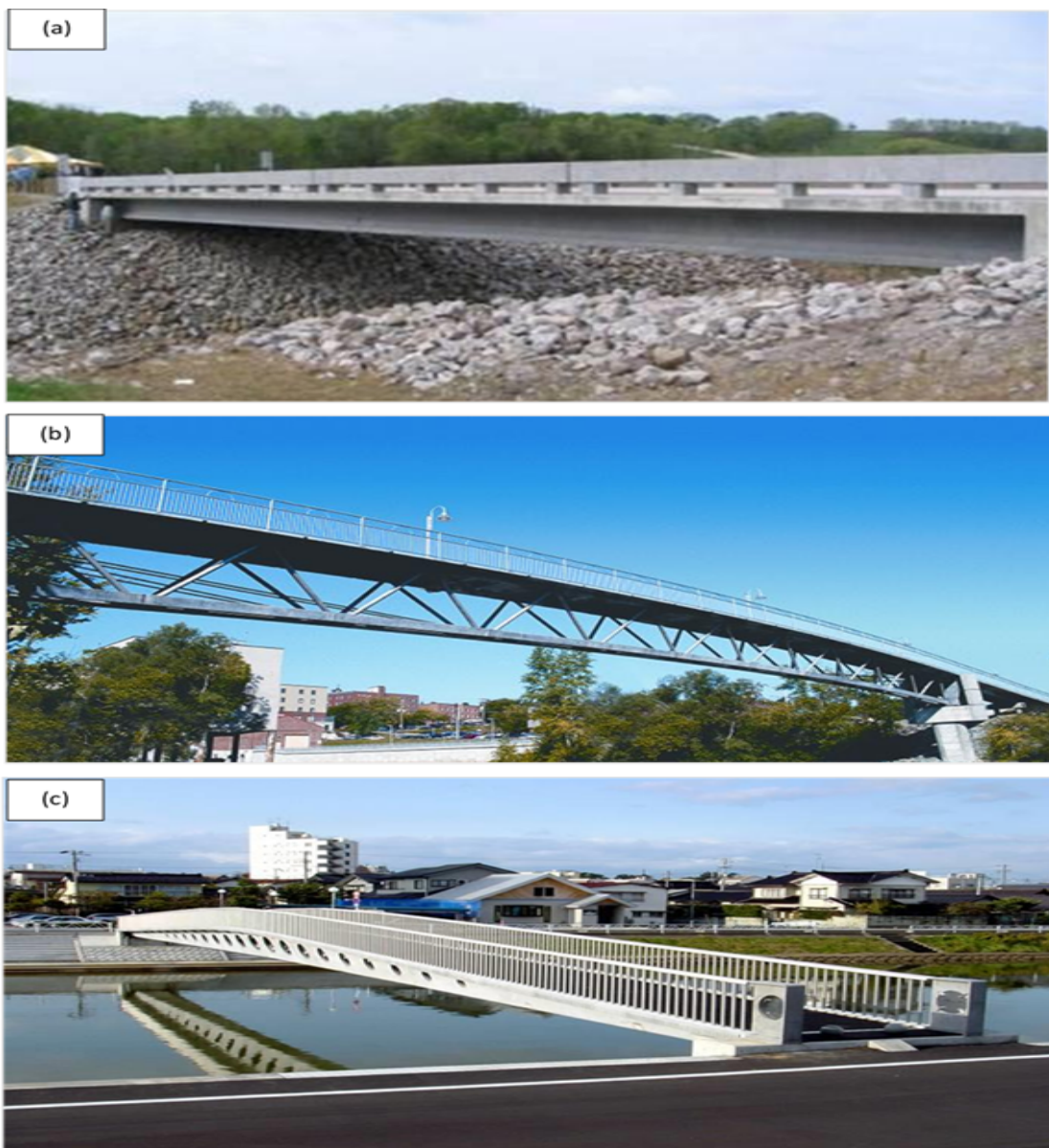
FIGURE 2.4: Repair of Bridges with UHPC (a) Mars Hill Bridge, Wapello County, IA (b) Sakata-Mirai bridge, Sakata, Japan (c) Pedestrian bridge, Sherbrooke, Quebec, Canada [22]
