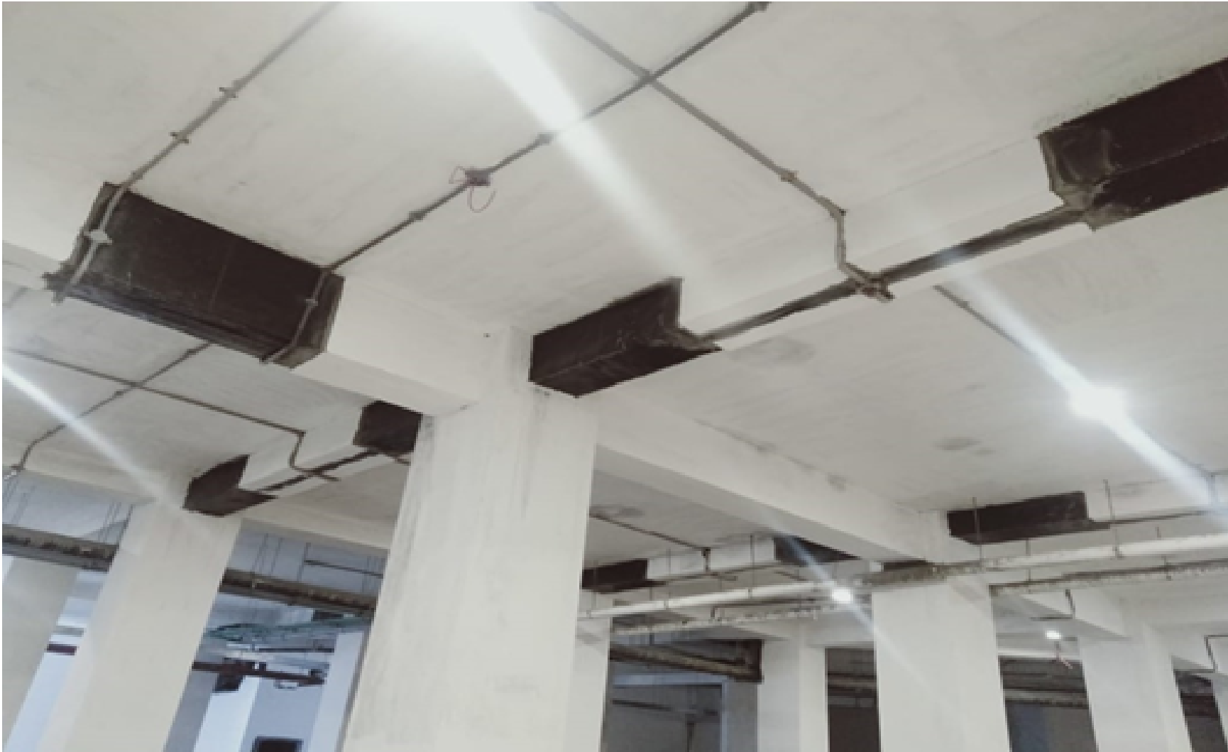
FIGURE 2.2: CRFP used to repair beams in a hospital at Rawalpindi Pakistan
