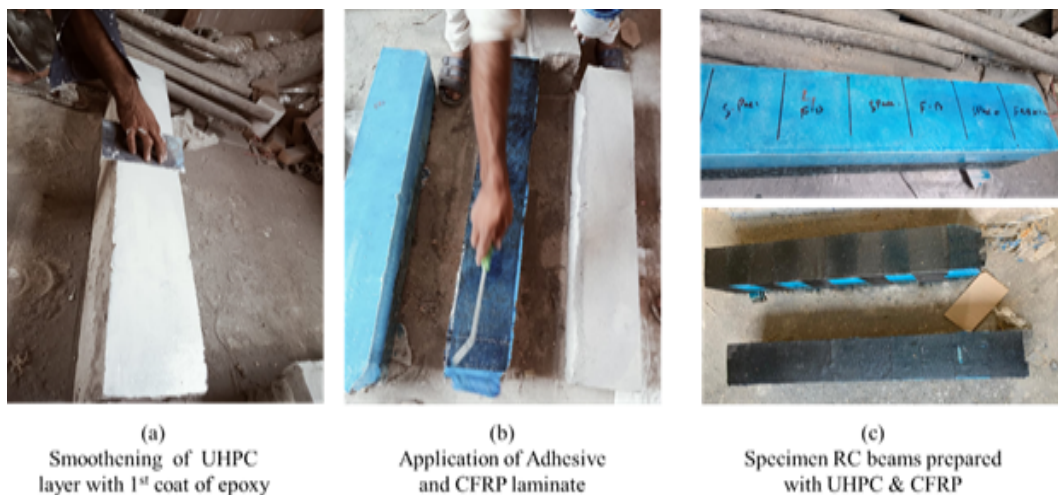
FIGURE 3.8: Application of CRFP Layer (a) Smoothing of UHPC layer with 1st coat of epoxy (b) Application of Adhesive and CFRP laminate (c) Specimen RC beams prepared with UHPC & CFRP
