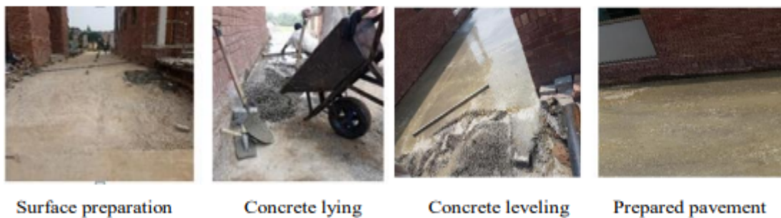
FIGURE 5.3: Wheat straw fiber reinforced concrete pavement [28]
